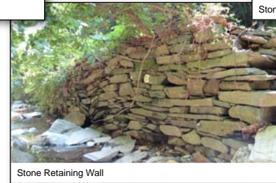
Stone Retaining Wall
