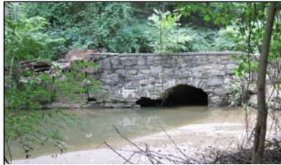
Soapstone Creek Culvert
