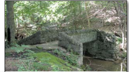
Stone Pedestrian Bridge
