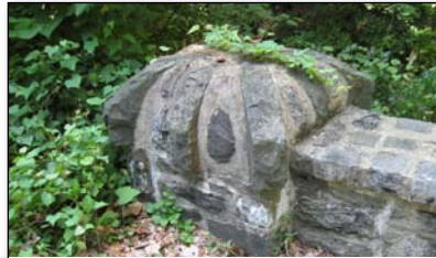
Grant Road Bridge Detail
